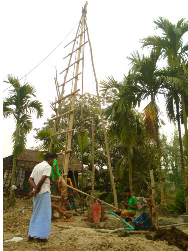
Figure 5 Drilling setup direct circulation method.
