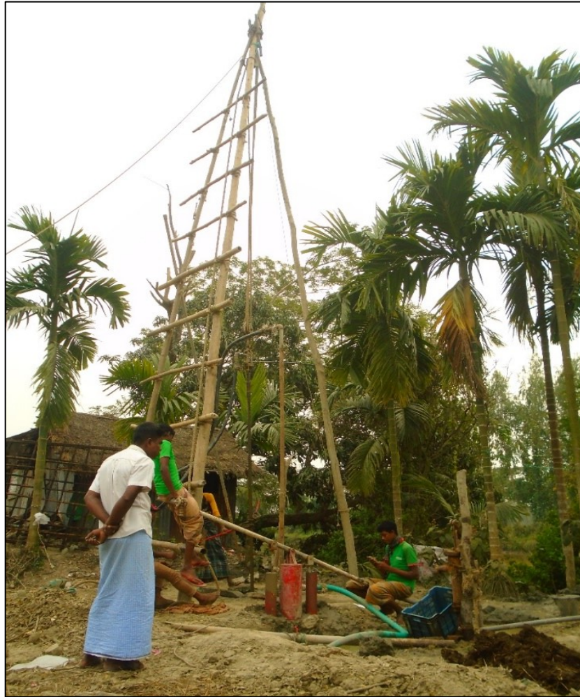
Figure 3 Drilling Procedure of Monitoring well (Source: CGR)
