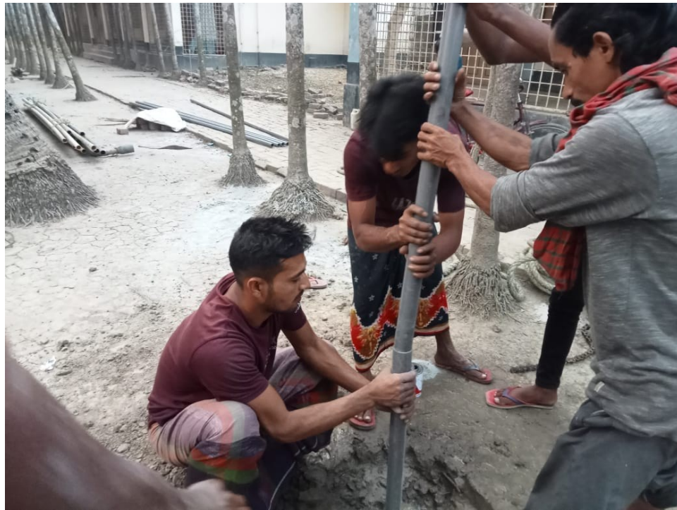
Figure 3 Installation of Monitoring Well in Mujibnagar Upazila
