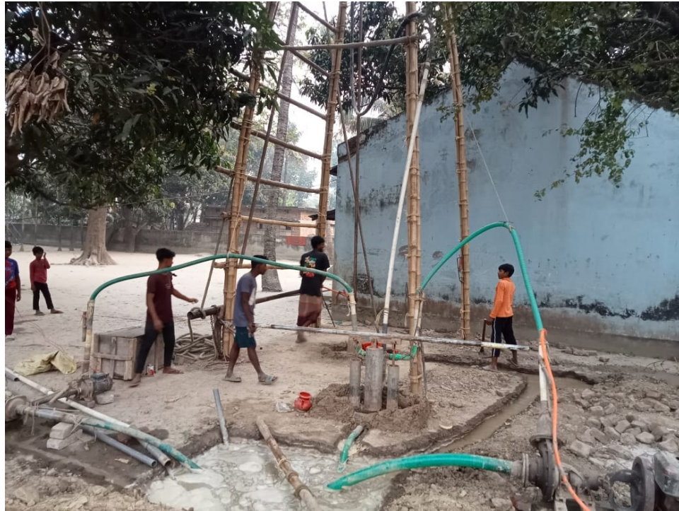
Figure 2 Drilling Procedure of Monitoring well in Mujibnagar Upazila.
