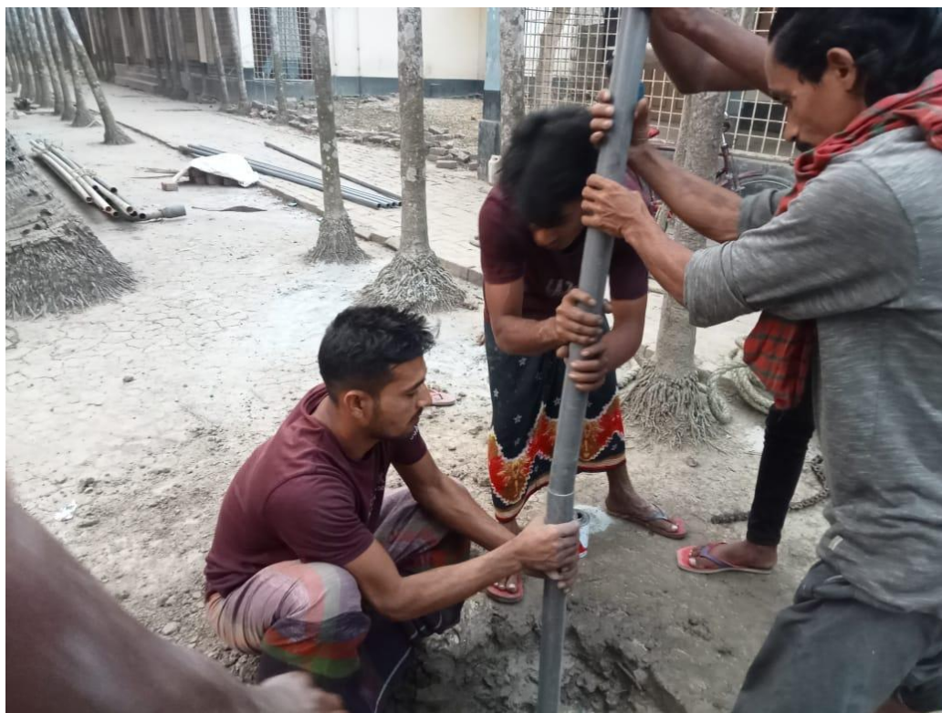
Figure 3: Installation of Monitoring Well in Mujibnagar Upazila
