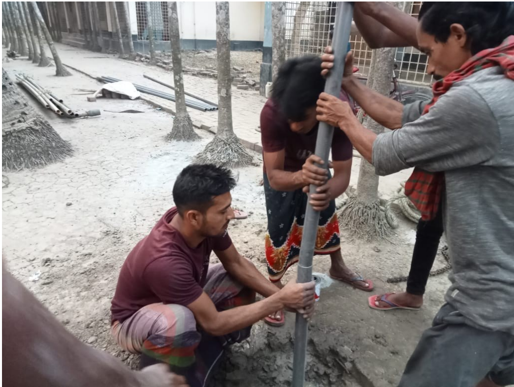
Figure 3: Installation of Monitoring Well in Mujibnagar Upazila
