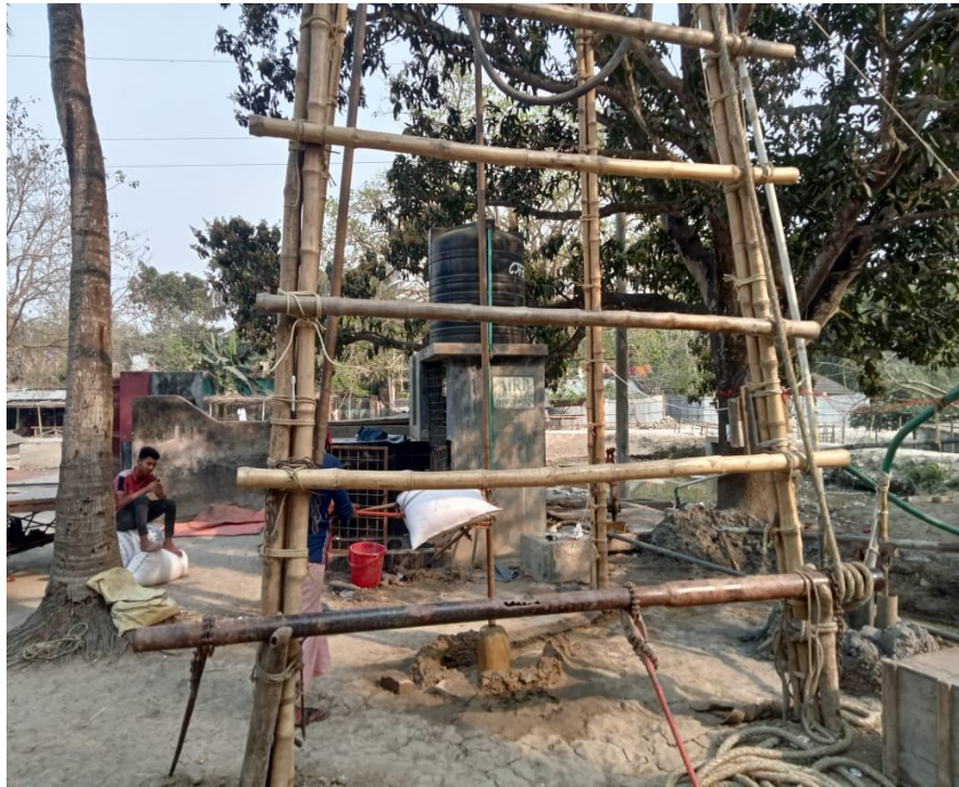
Figure 2: Drilling Procedure of Monitoring well in Mujibnagar Upazila.
