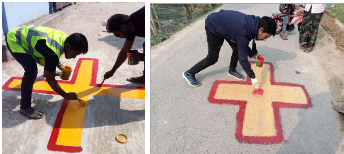
Figure 5-2: GCP marking on the ground according to the GCP plan before drone survey
