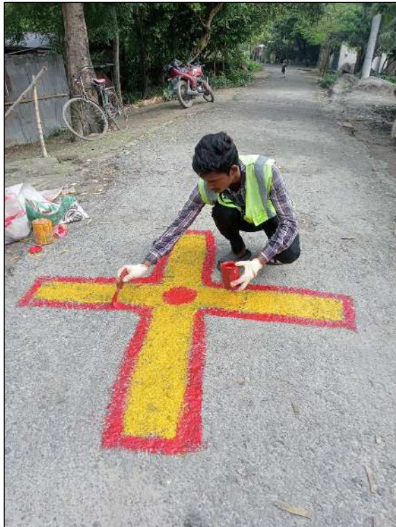
Figure 3-4: GCP Marking on Ground As per GCP Plan Before Drone Survey
