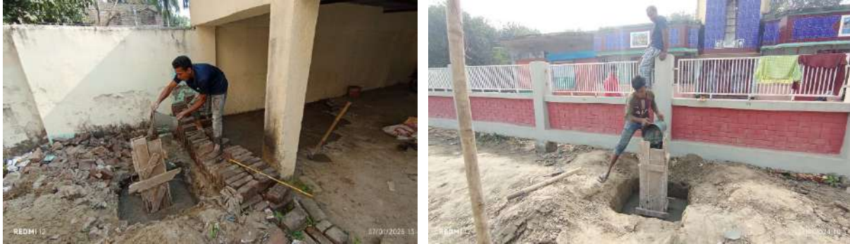
Figure 2-3: BM Pillar establishment in the project area
